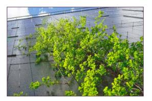
Greenery integration on shopping centres is easy. The façade face selected for the integration should in principle be blind. It should face NE-SE and NW-WE. The free-soil surface should be available at the wall bottom (or some bowls on the pavement should be considered). That would allow to get installation and maintenance of plants feeding as more natural.
